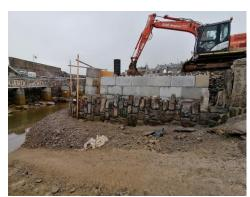
Well not a lot has changed since the last chat. Although work on the walls have continued and facing is well above the water line on the railway pier as well. Placing the capping stones on the east pier appears to
